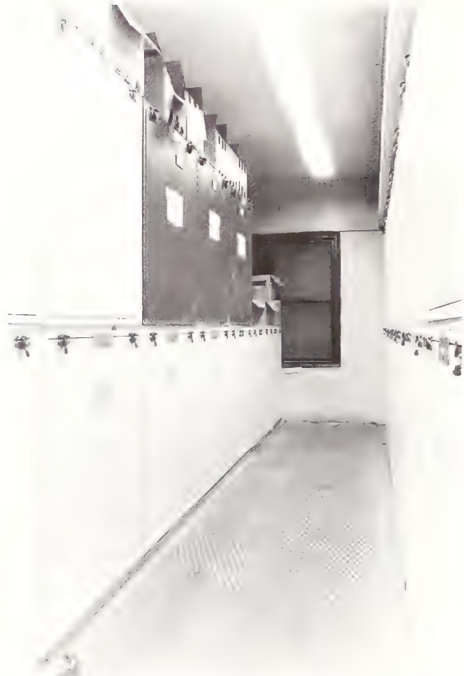
East range ground floor, April 1984, showing the steel decking and windows that open onto the corridor but are plastered-over on the exterior. From the 1930s to the 1960s, vertebrate fossils were stored here. The cases, covered to keep out dust, now contain invertebrate fossils; the fluorescent lights are moderately new. The Scanning Electron Microscope Laboratory is directly below.
